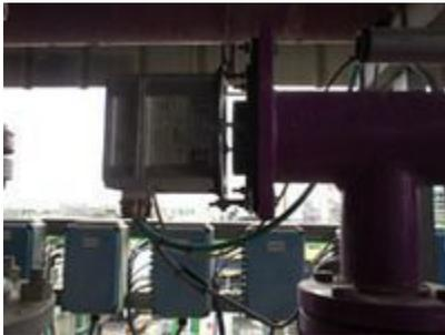
The SafEye Duct Mounted Gas Detector uses its source and detector to detect gases at the 3.4m wavelength with the ability to determine the concentration of the gases, before they reach explosive levels. Relevant precautions can then be taken to ensure that an explosion doesn't occur.
